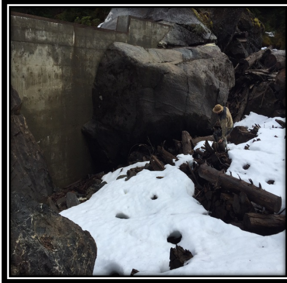
Tyee Lake Weir Right Abutment 2016
