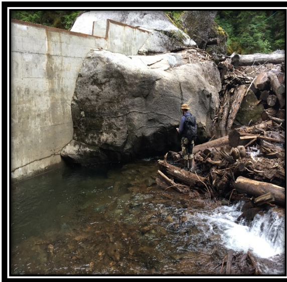
2015 Upstream Weir Right Abutment
