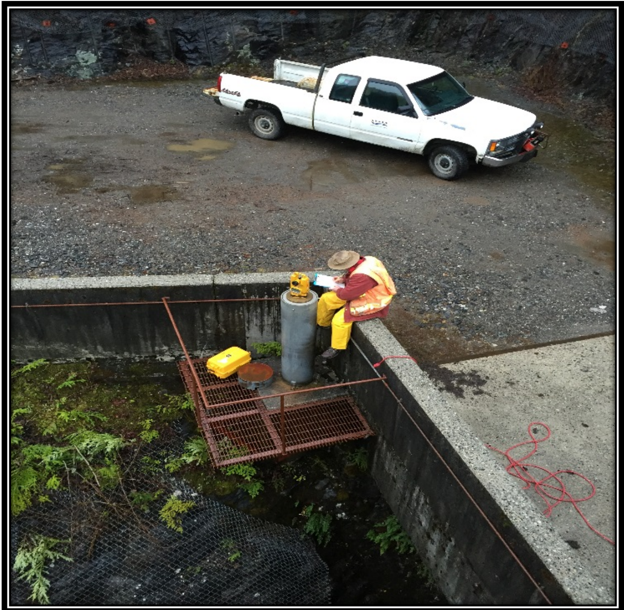
Swan Lake Dam Settlement Survey
