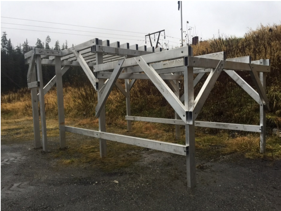
Satellite Dish Platform
