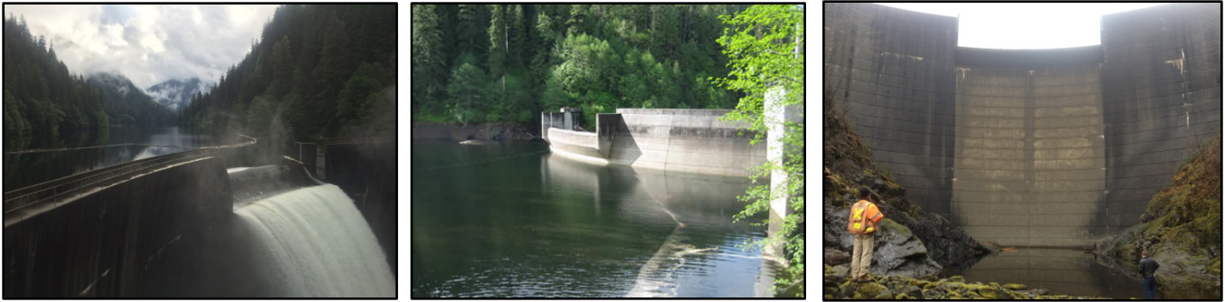
Three perspectives of the Swan Lake Dam and spillway as it appears today.
