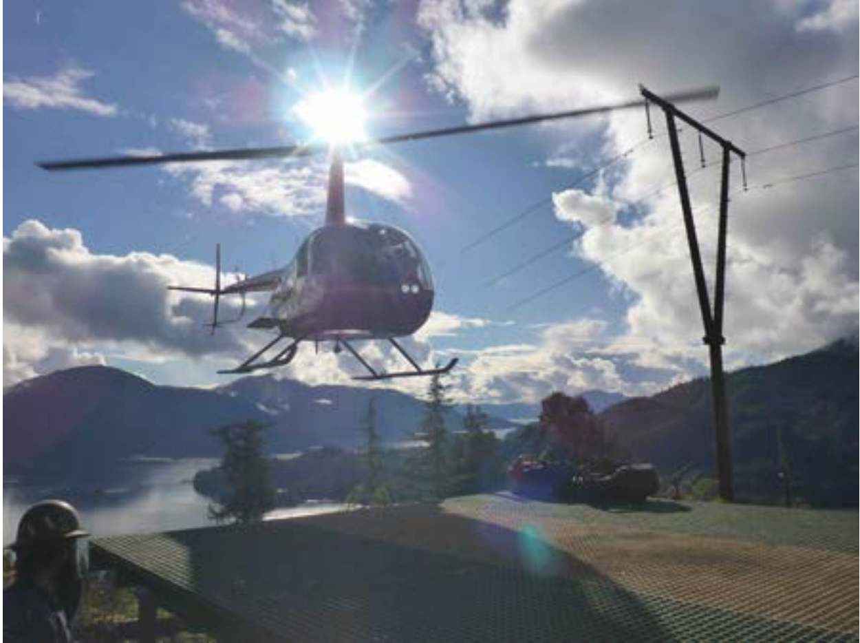
New Helipad at Tower 97 on the Intertie
