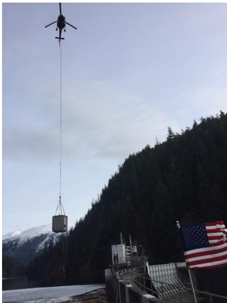
Compressor Building Placement
