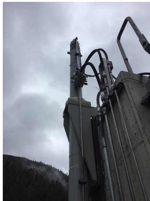
FWG Hydraulic Lifting Cylinder
