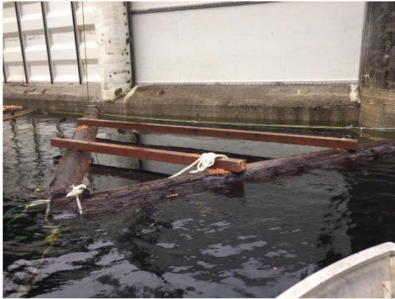
FWG A-Frame Debris Deflector
