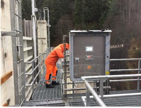
FWG Control Panel - Located at Gate
