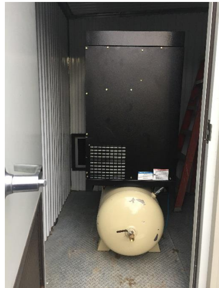
Compressor Placed in Building
