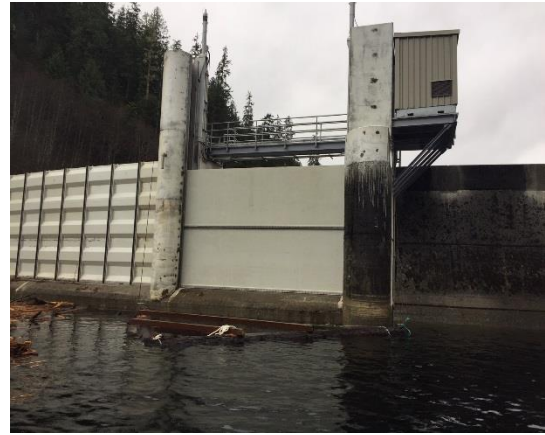
FWG A-Frame Debris Deflector
