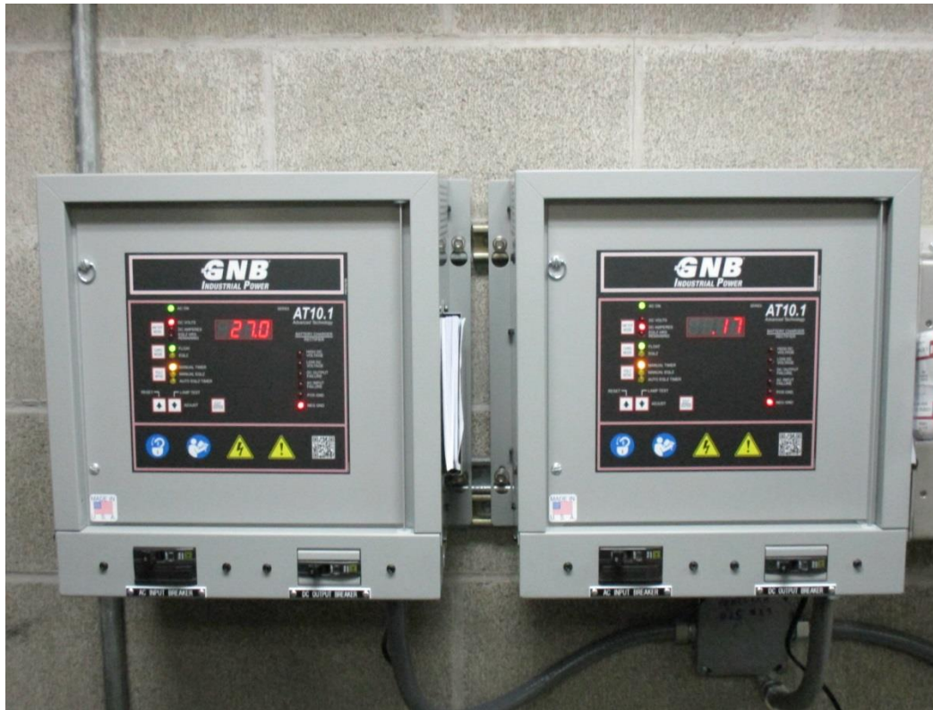
Above: New install of diesel generator PLC battery chargers. Below: SEAPA's new valve house emergency generator
