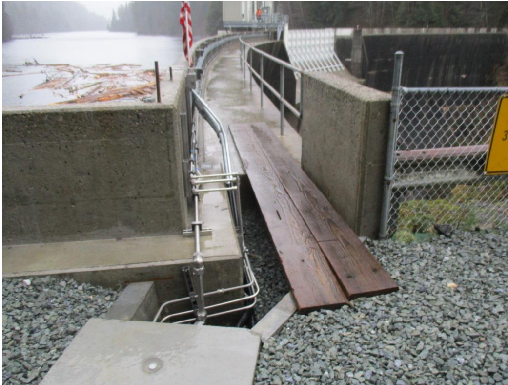
Above: Gate hydraulic lines exposed. Below: Fabrication of protective plates & covers.
