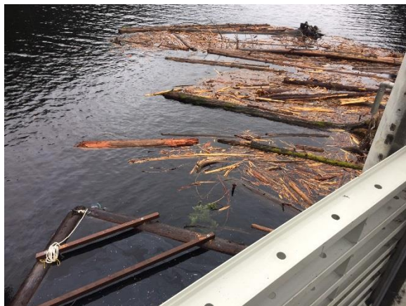
FWG A-Frame Debris Deflector
