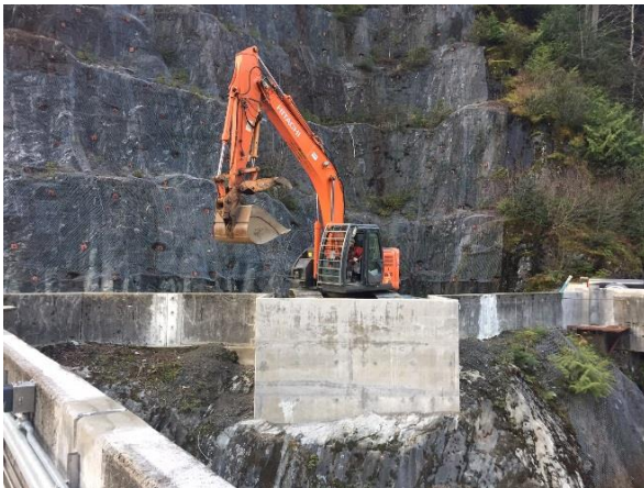
New Debris Removal Platform
