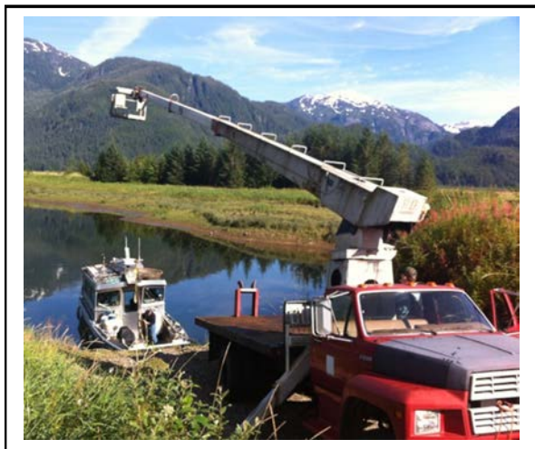
Unloading propane tanks at Tyee project.
