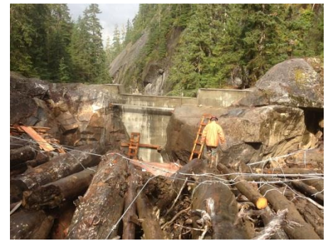
(Tyee weir, upstream side)
